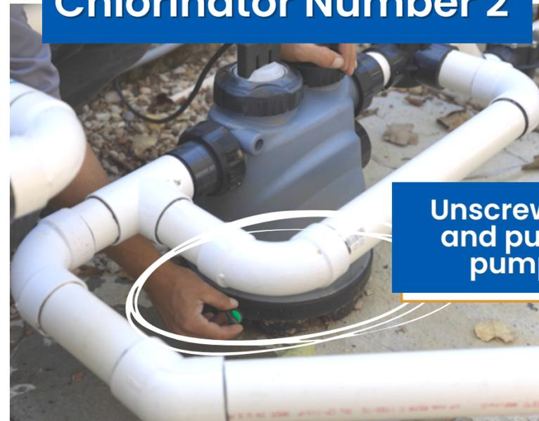
Unscrew drain plug and put into main pump basket.
