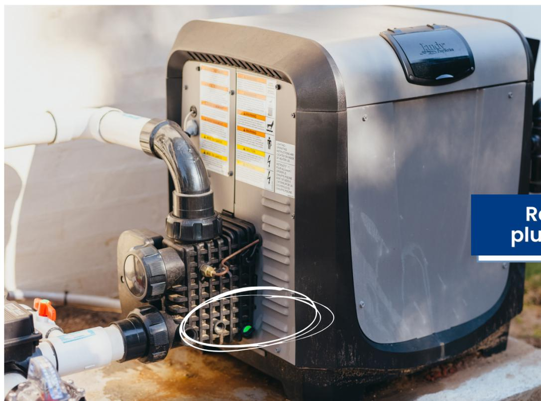
Remove drain plug from heater
