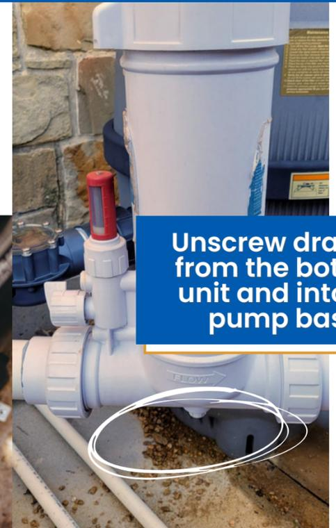
Unscrew drain plug from the bottom of unit and into main pump basket.
